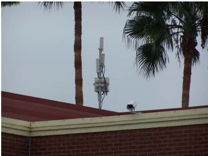
[CAPTION] CCTV cameras are connected via eight Azalea MSR2000 and two MSR4000 routers, providing a cost-effective solution to provide the mall with wireless video surveillance.
